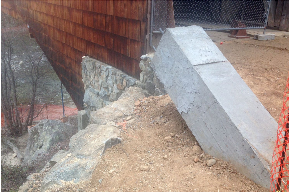
Photo No. 5 Tension anchor for interim stabilization
