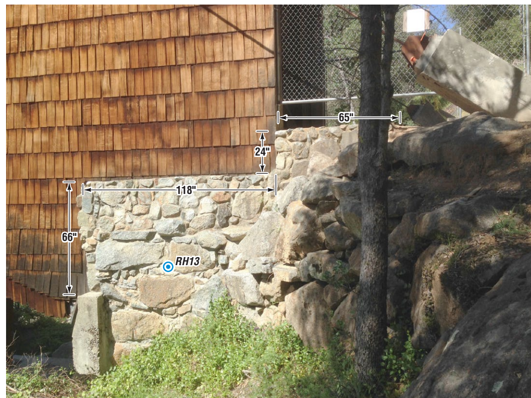
Upstream Abutment Profile
