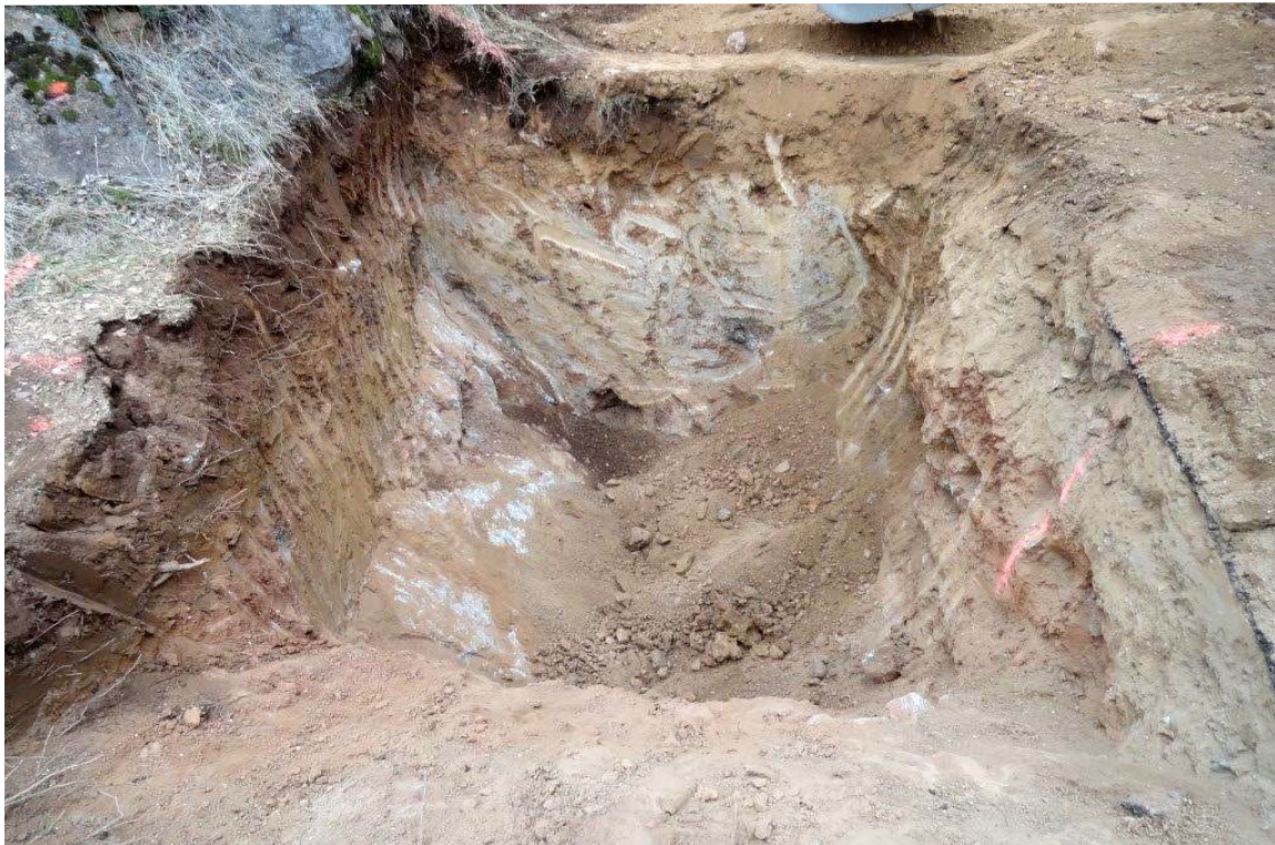
Photo No. 8 Typical subsurface conditions – north abutment area
