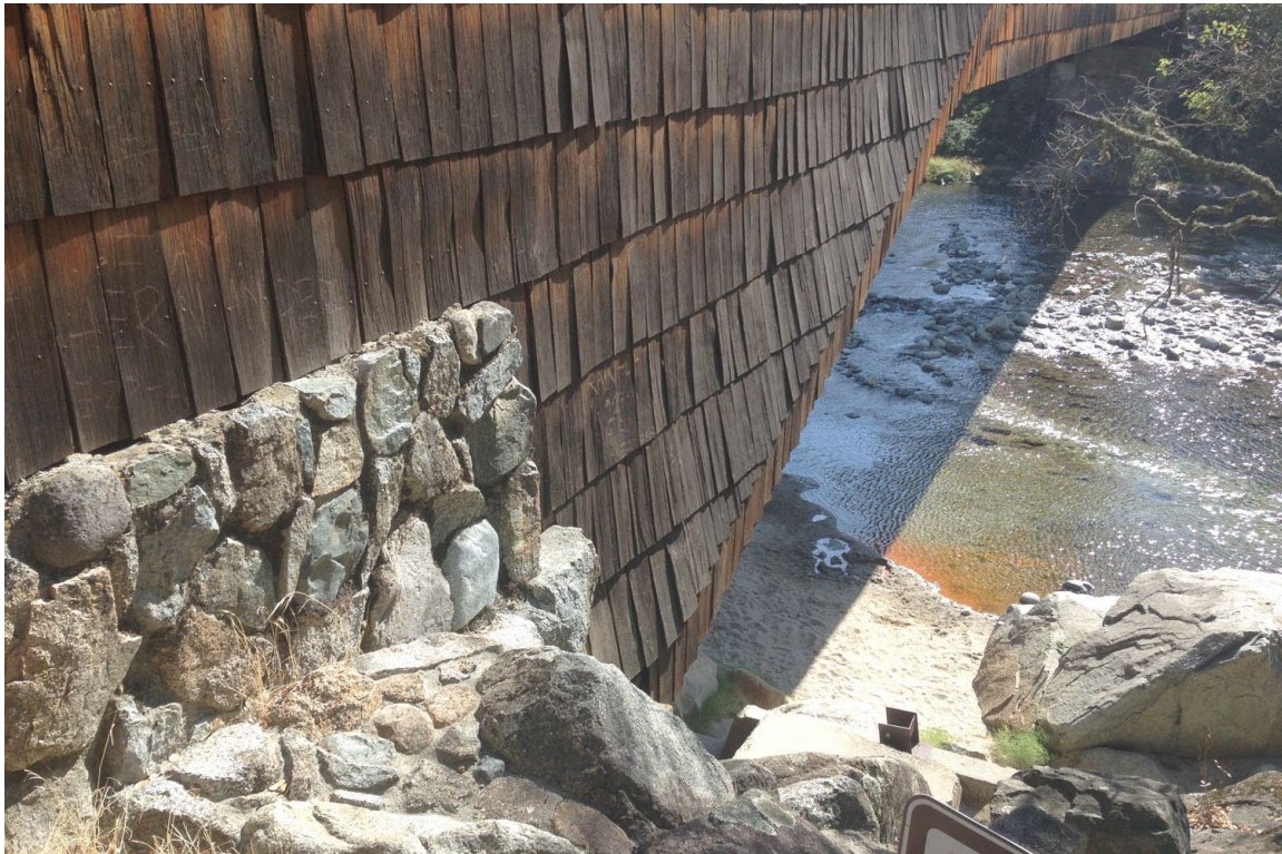
Photo No. 1 Existing bridge as viewed from north to south
