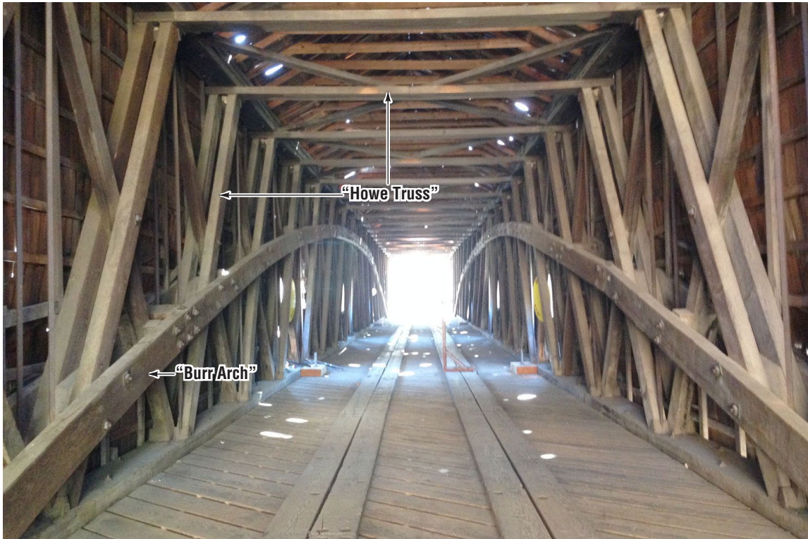
Photo No. 3 Bridge interior
