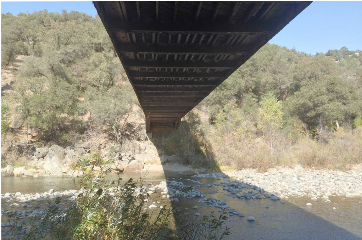
Photo No. 2 Existing bridge as viewed from below, south to north
