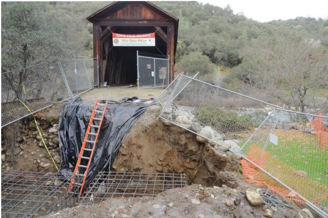
Photo No. 6 South tension anchor footing
