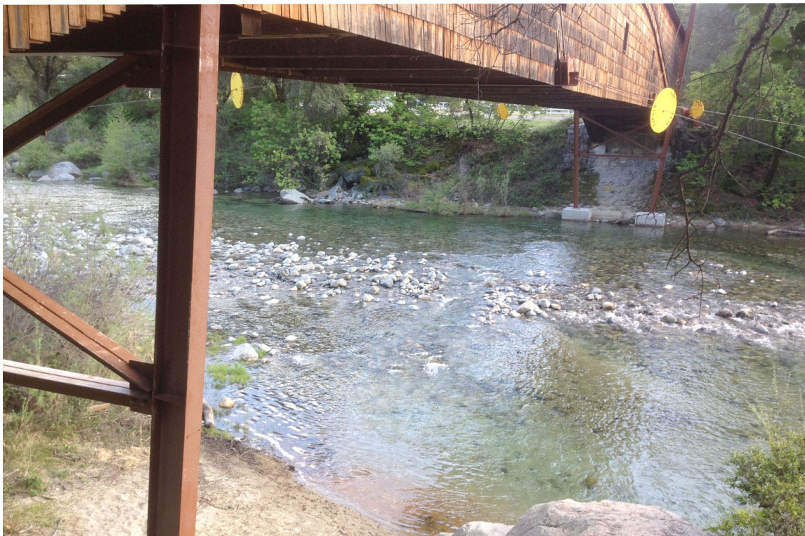
Photo No. 4 Interim stabilization piers
